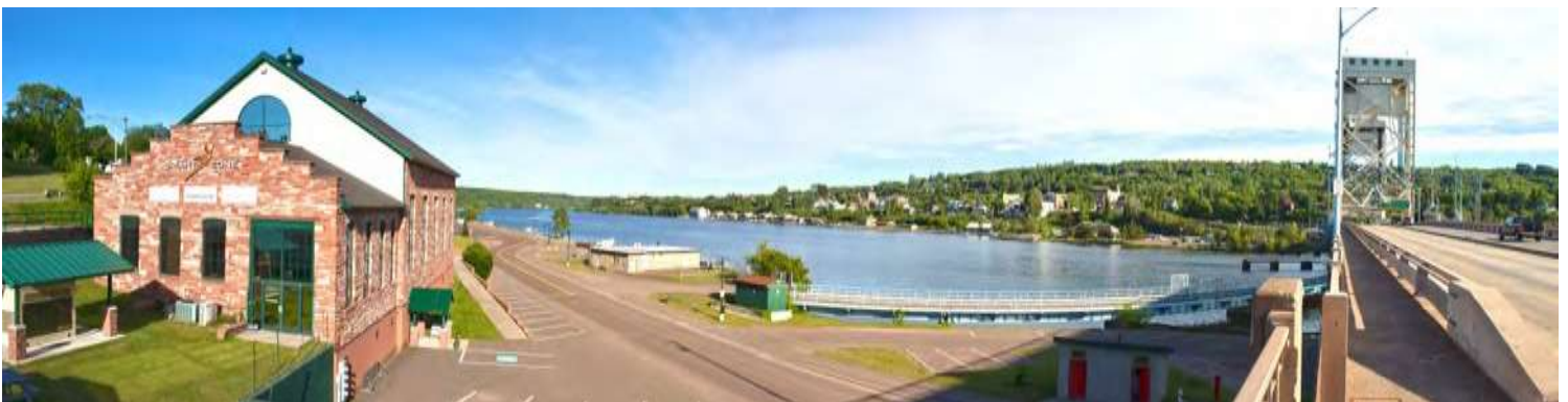
MTEC SmartZone Powerhouse, Houghton, Michigan
