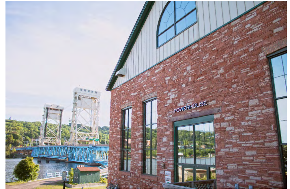
Powerhouse in Houghton
